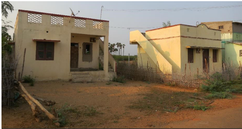
Figure 4: Photo of to-scale model houses in Tarangambadi, Tamil Nadu. House design took account of local livelihood needs, in this case having an accessible flat roof so fishing families had space to dry fish.
