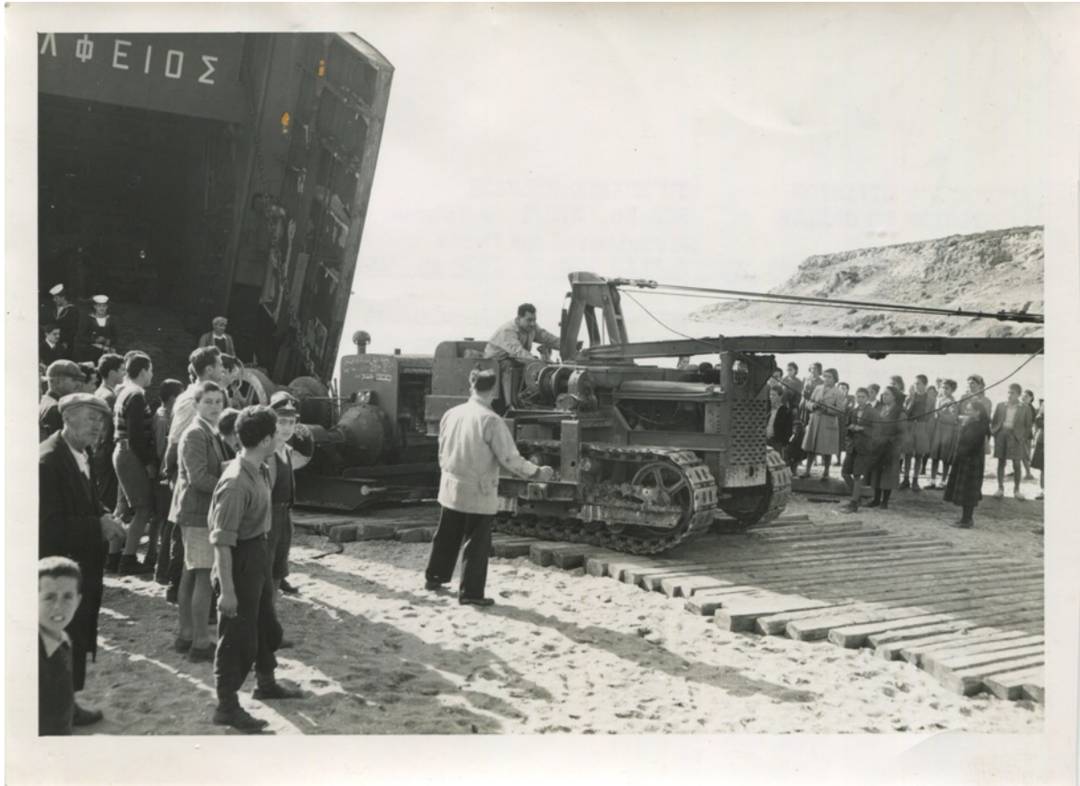
Figure 133. Arrival of construction machinery at Aliveri, Evia. Unknown photographer. 1951. ELIA-MIET.
