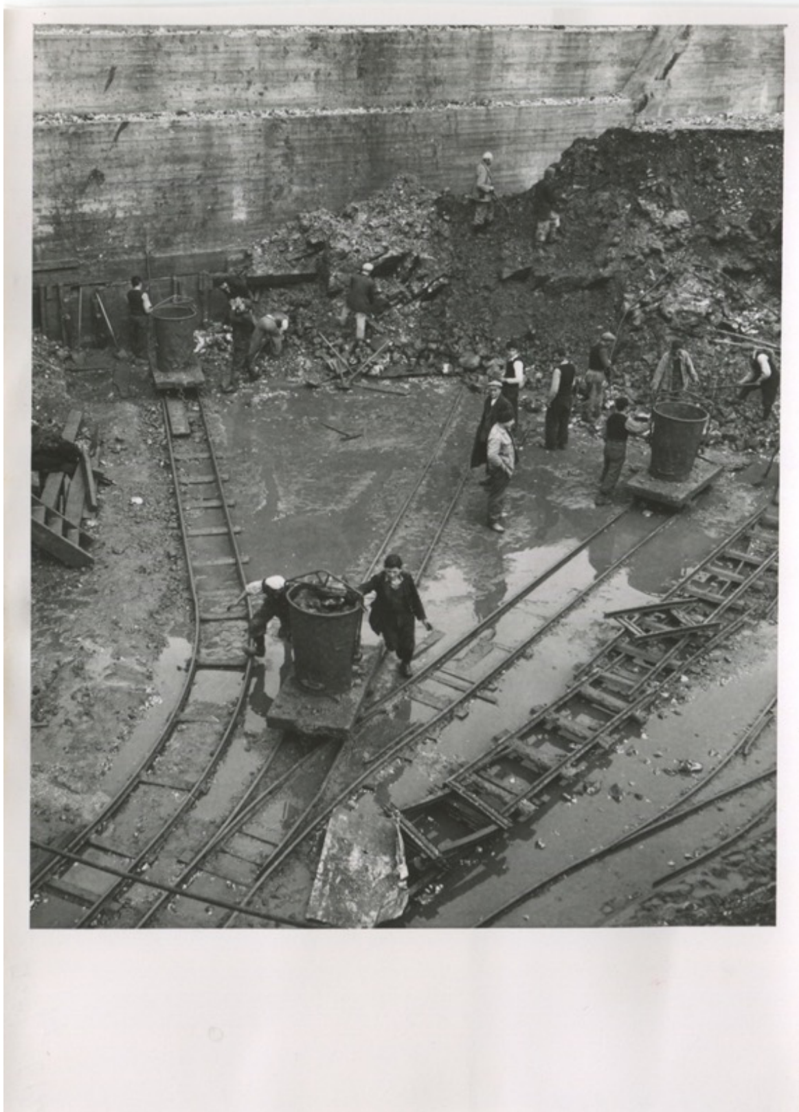
Figure 141. Construction of dam at the Louros river, Epirus. Unknown photographer. 1953. ELIA-MIET.
