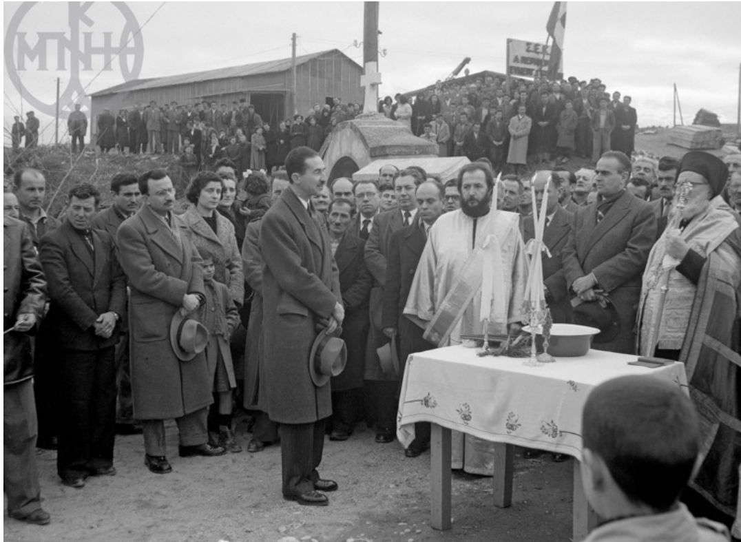
Figure 52. Ground breaking ceremony for railroad works, with Konstantinos Karamanlis, Minister of Public Works and Transport, in attendance. Ioannis Lampros. 1950s. Benaki Museum.
