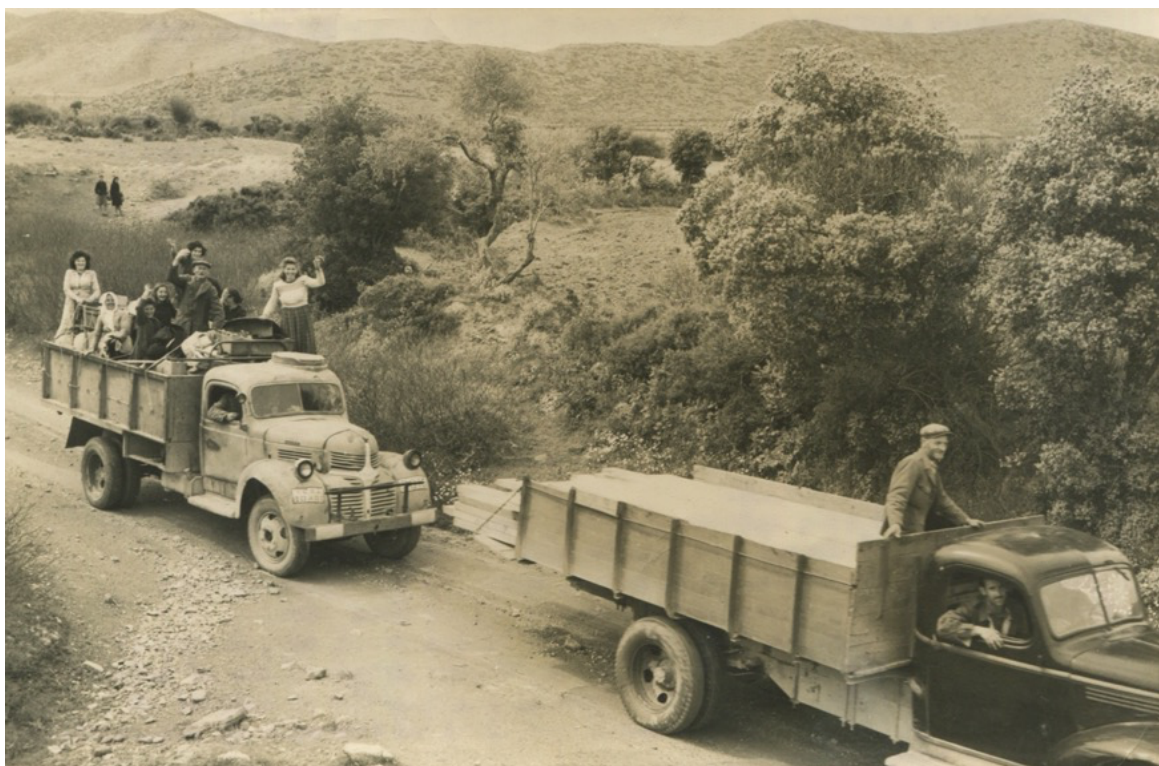
Figure 123. Trucks with lumber 'bought with Marshall Plan funds' and returning villagers. Unknown photographer. 1950. ELIA-MIET.
