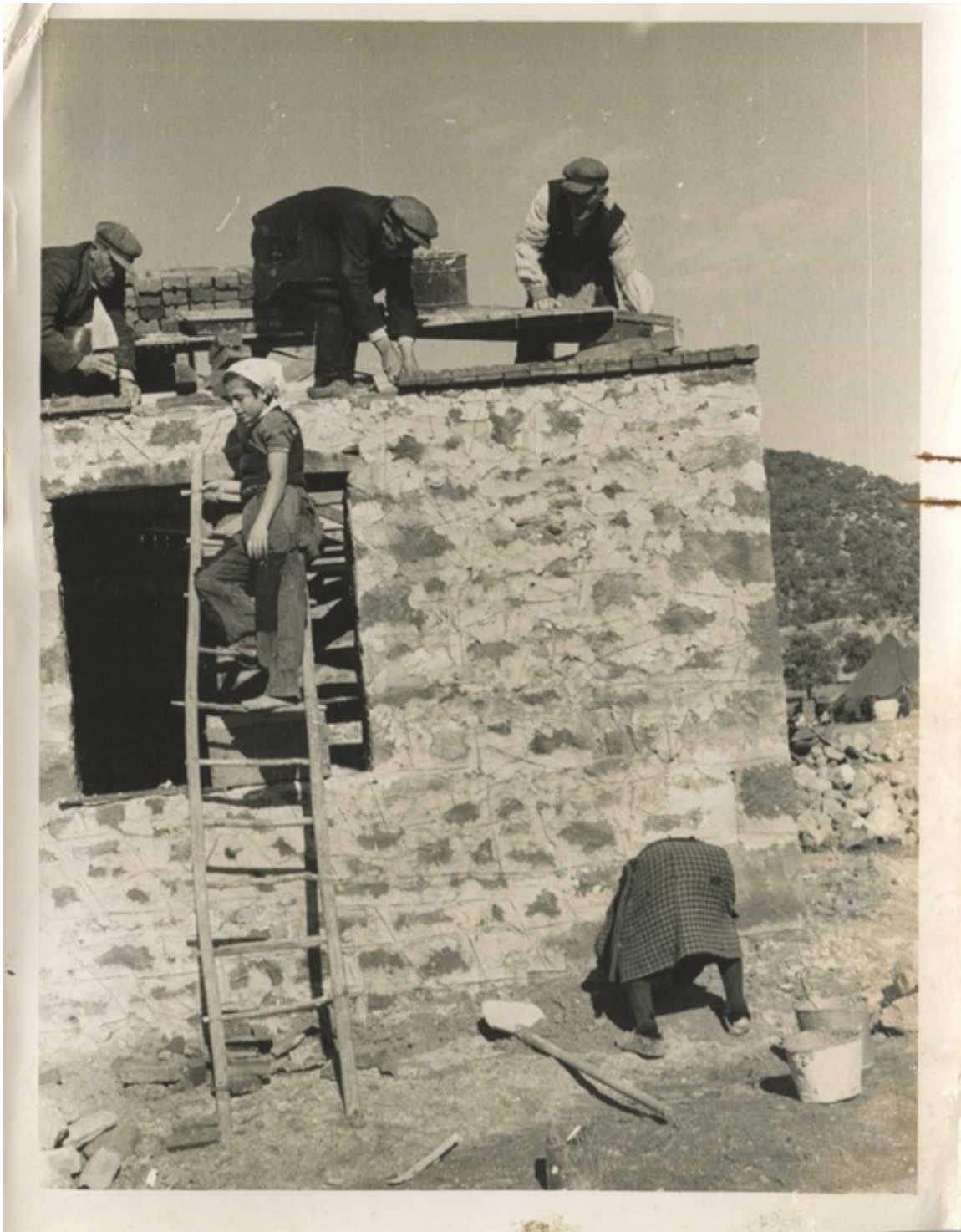
Figure 128. Families building homes in Nipsa. Unknown photographer. 1950. ELIA-MIET.
