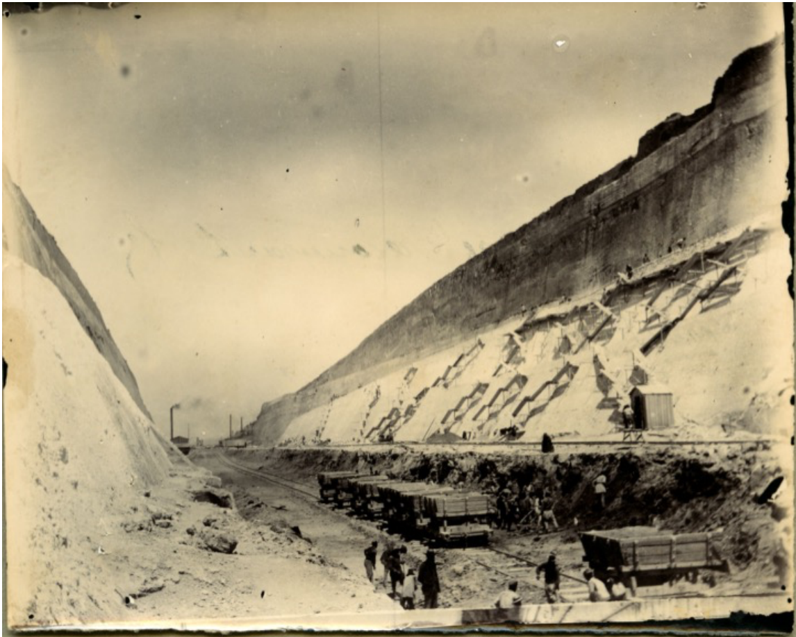
Figure 13. Construction of the Corinth canal. Unknown photographer. 1880s. BNP Paribas.
