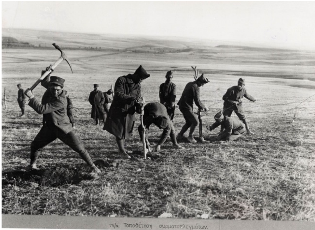
Figure 26. Erecting barbed wire. Unknown photographer. March 1921. EIM.
