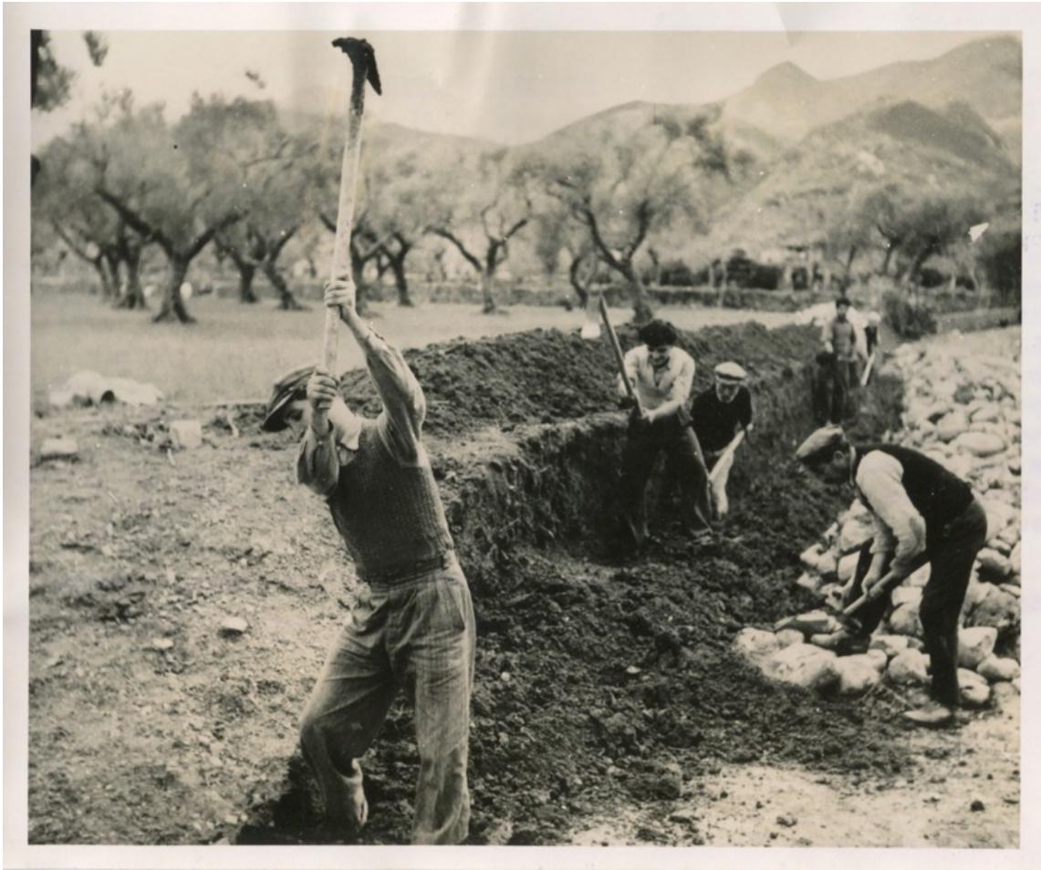
Figure 129. Villagers of Paleopanaghia laying the foundations of the new road. Unknown photographer. 1951. ELIA-MIET.
