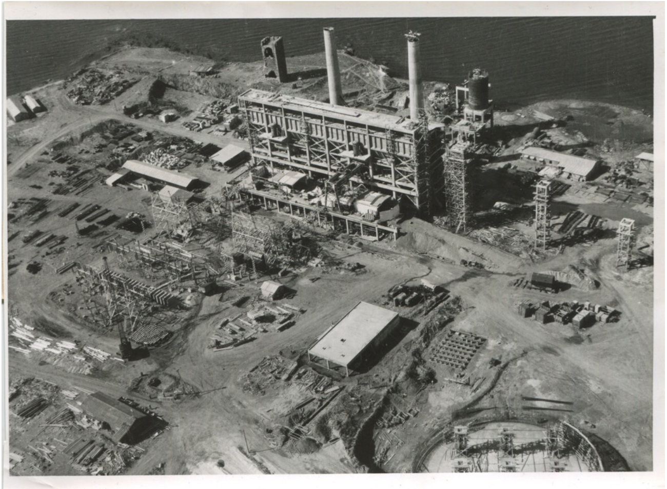
Figure 136. Aerial view of the Aliveri power plant. Unknown photographer. 1953. ELIA-MIET.
