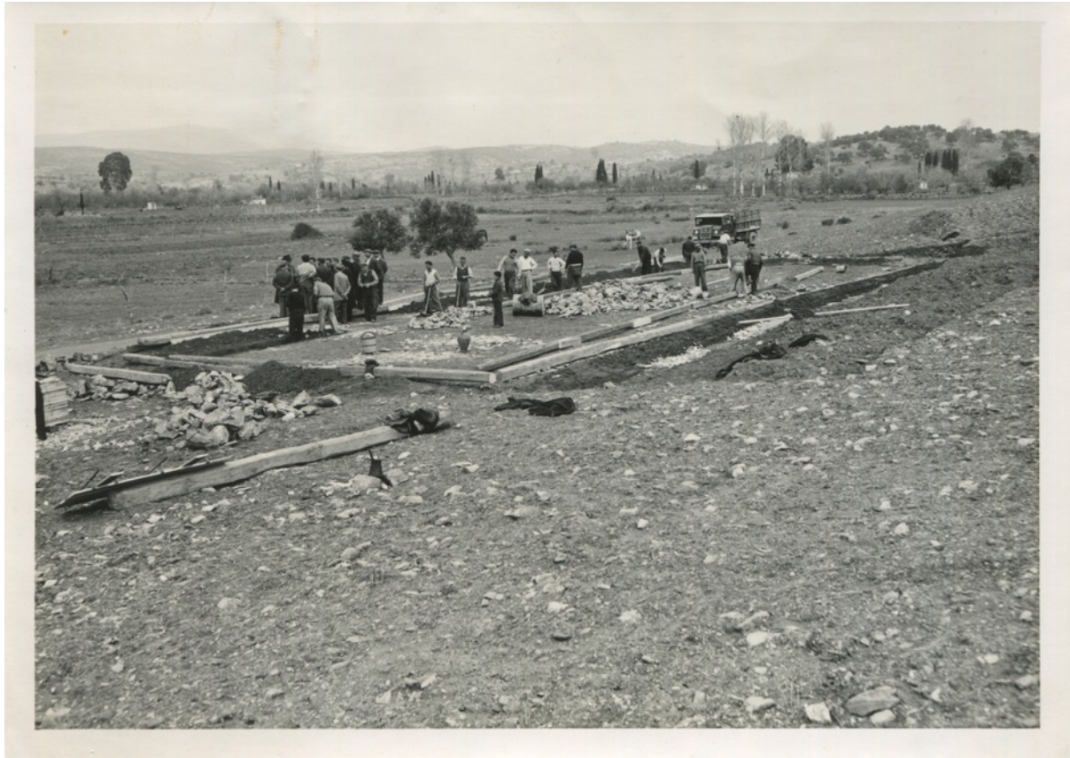
Figure 135. Warehouse construction at Aliveri. Unknown photographer. 1951. ELIA-MIET.
