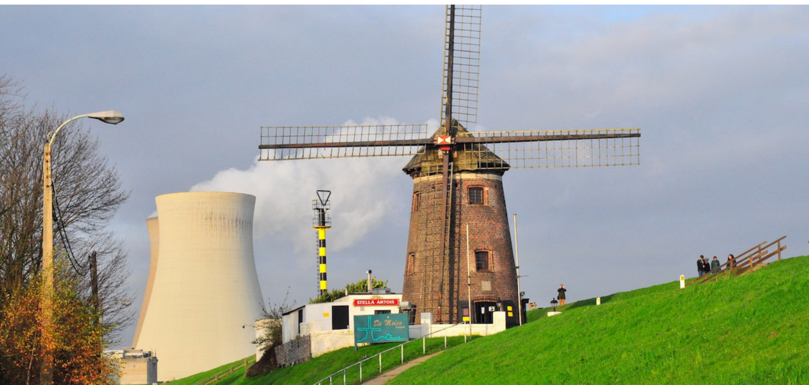
THE DOEL NUCLEAR POWER PLANT COPYRIGHT: BOUDEWIJN HUYSMANS
