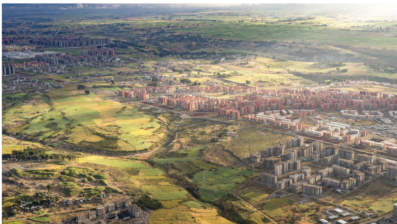
Image 2.1 Urban and industrial construction site in Addis Ababa. Source: Shutterstock
