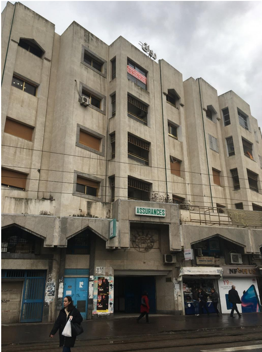
Fig. 23: Galerie 7 from Avenue Habib Thameur, April 2021
