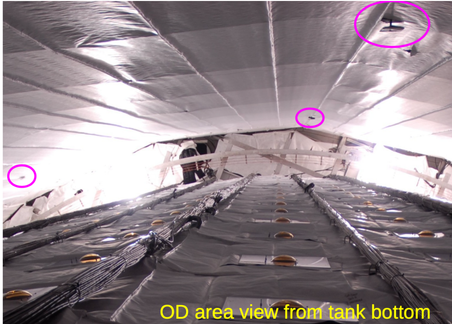
Figure 4.14: Photo taken in the OD barrel region showing a few protruding fibre tips (circled in pink) [107]. Visible at the bottom of the image is the steel structure that supports the OD PMTs on one side, as seen in the photo, and the ID PMTs on the opposite side, which are not visible. The ID volume is located behind this wall.
