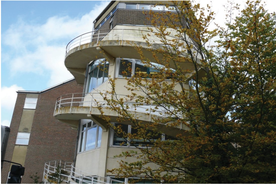
FIGURE 8 South-facing Nightingale wards with curved fire escapes at Kent and Sussex Hospital (surgical ward shown at level 3).
