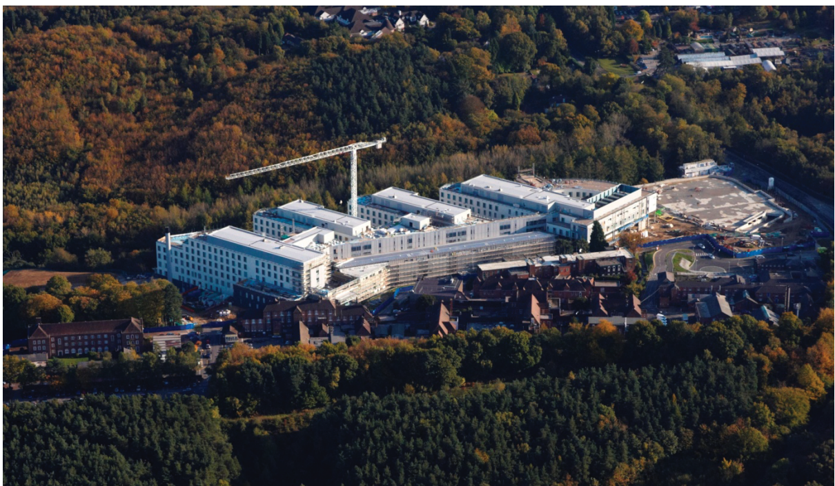
FIGURE 1 New hospital during construction: old Pembury Hospital in the foreground.
