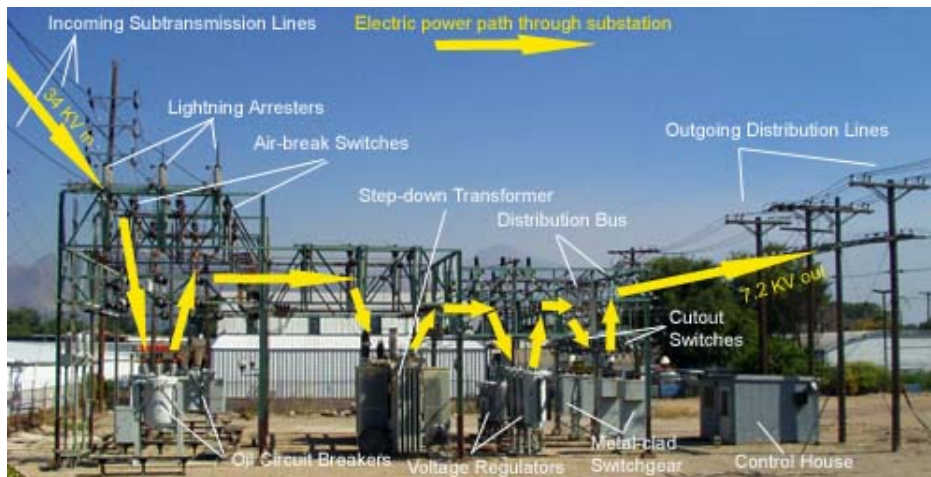
Figure 2.6: Energy flow through a typical substation. Credit-OSHA.
