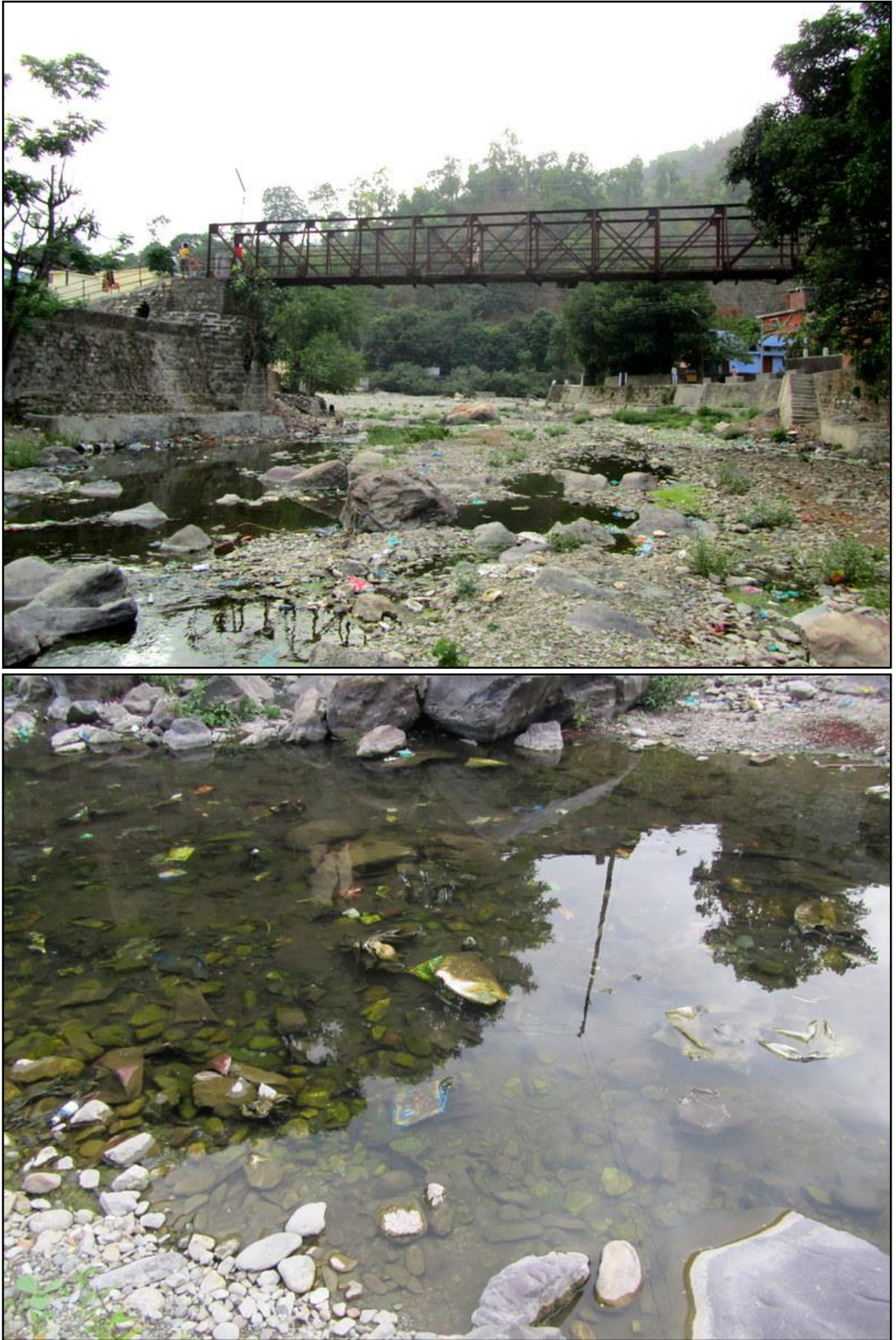
Figure 2.6.3: Photographs showing the unprotected reaches of Khoh River (PHOTO: N. Gupta).
