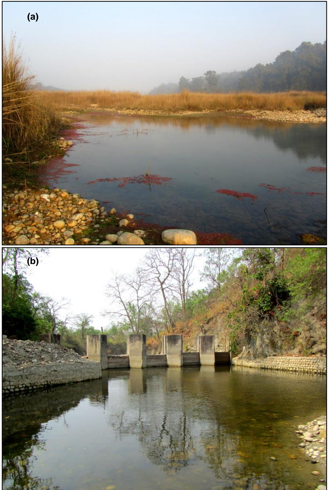
Figure 2.7.5: Photographs showing (a) an impoundment, and (b) a weir within Rajaji national park to provide water for park animals (PHOTO: N. Gupta).
