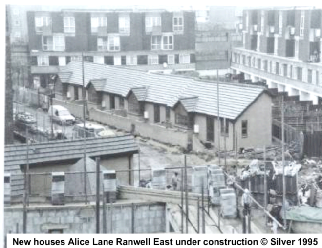
Figure 6.9 Construction of Alice Lane
