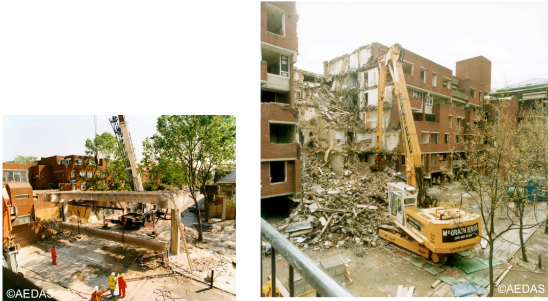
Figure 8.3 Demolishing the walkways
