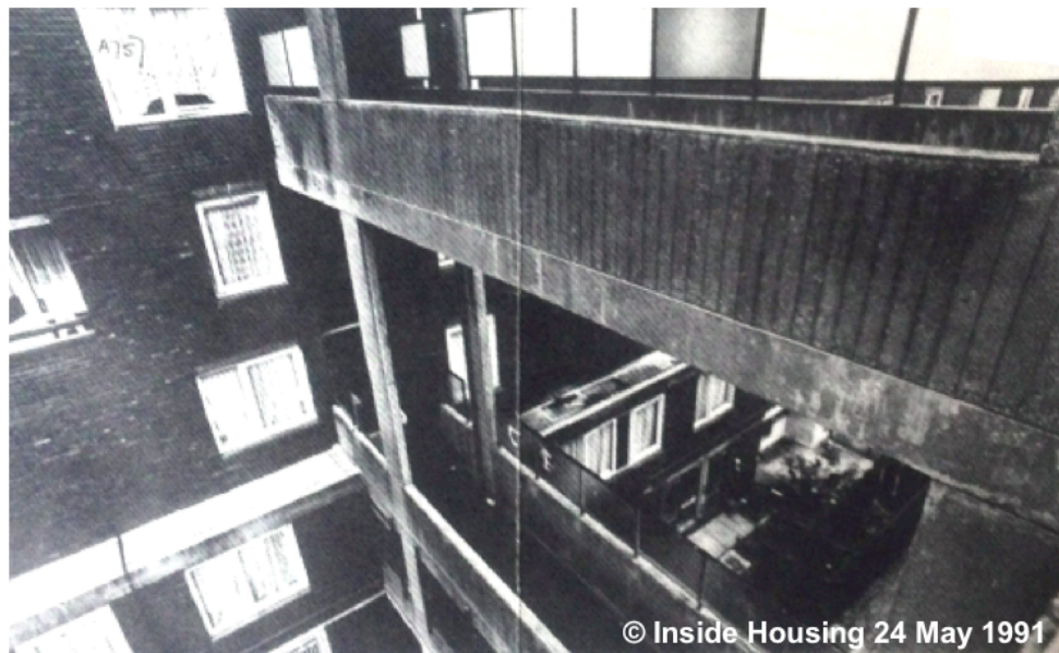
Figure 6.8 Walkways at Ranwell East Estate
