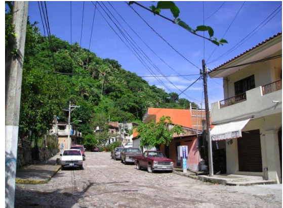
Photo 4.15 Project A Location
