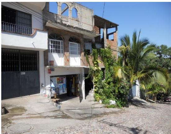
Photo 4.16 Project A Location
