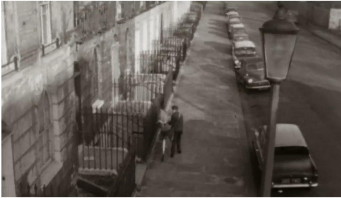
Figure 4.11: Pre-gentrification houses in Gibson Square, note the facades in disrepair. ( Home Stories by Channel 4 (2001)).
