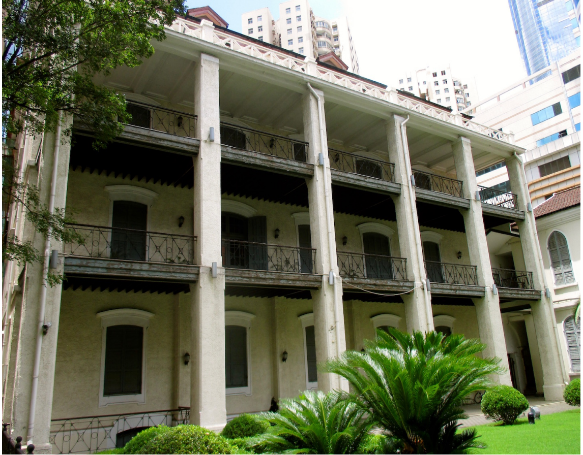
Fig. E.3. Exterior of the Xujiahui Library.
