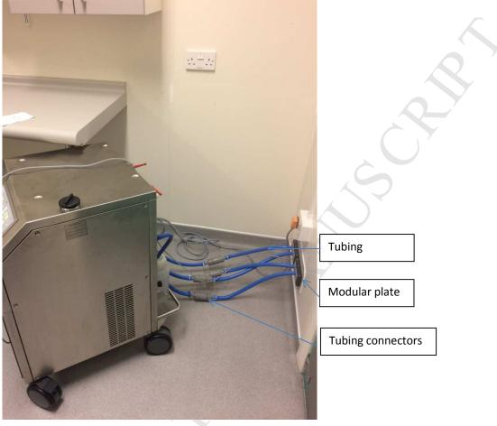
Figure 7. Position of the tubing through the wall into the operating theatre, using antislip matt housing and connection to the cardiopulmonary bypass equipment.
