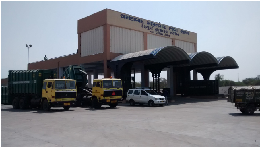
Figure 3: Transfer station, Ahmedabad Municipal Corporation (AMC) (Source: Author's photo)
