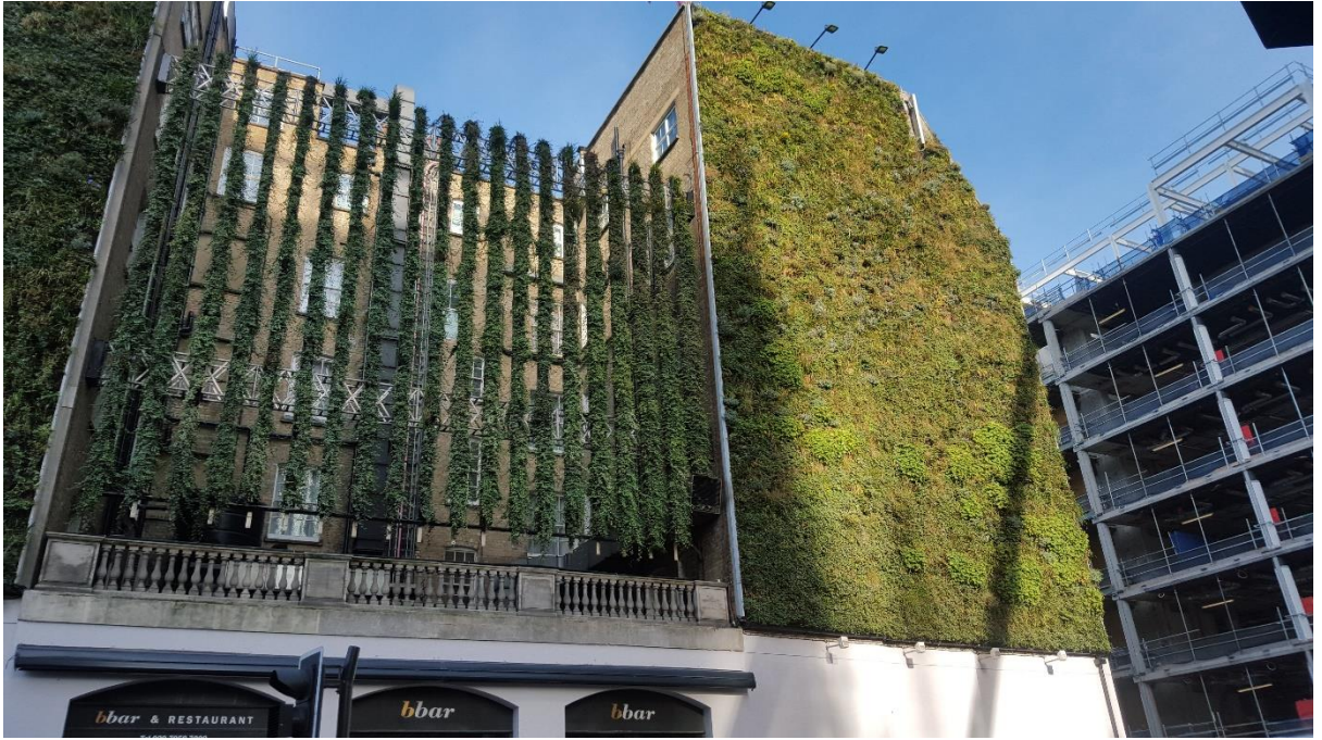
Figure 6.7 Living wall on the side of The Rubens at the Palace Hotel, in Victoria BID area (Source: Author)
